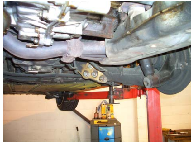
Adjustment points all cleaned and lubricated
